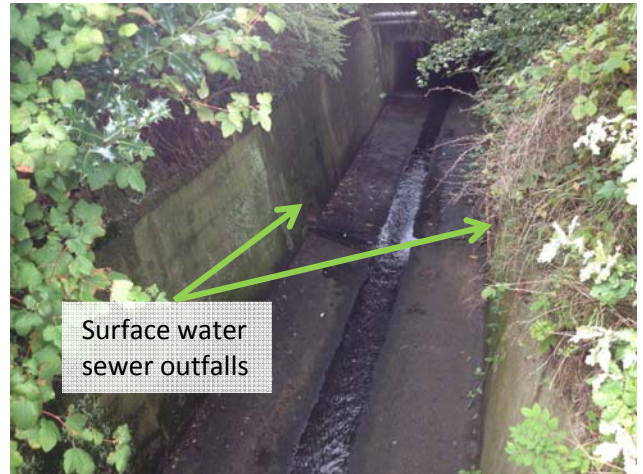
Photograph 3-7: Surface water outfalls to the tributary of Prittle Brook
