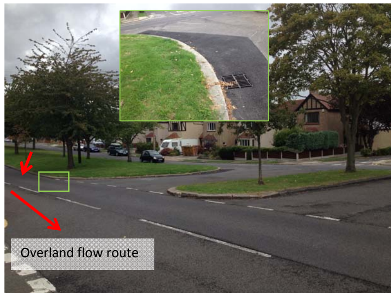
Photograph 3-5: Crossing at Highlands Boulevard at the junction of Adalia Crescent and Walker Drive (looking south). Detail of new gullies.
