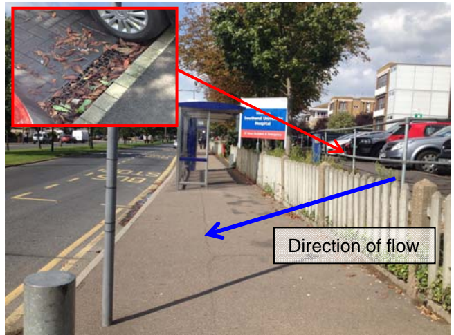
Photograph 3-2: Car park and Prittelwell Close (looking west) including detail of car park drainage
